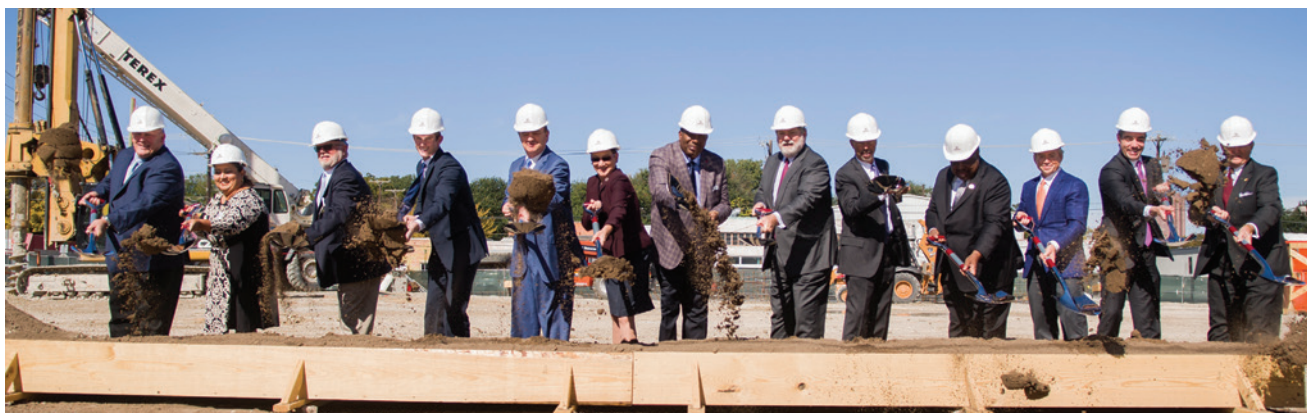
Texas A&M representatives, state elected officials and other dignitaries turn dirt at a mid-morning site dedication attended by hundreds of students, faculty, staff and friends. With Nussbaumer Street closed to traffic, a 180-foot tent accommodated a stage, seating and catered barbecue lunch.
